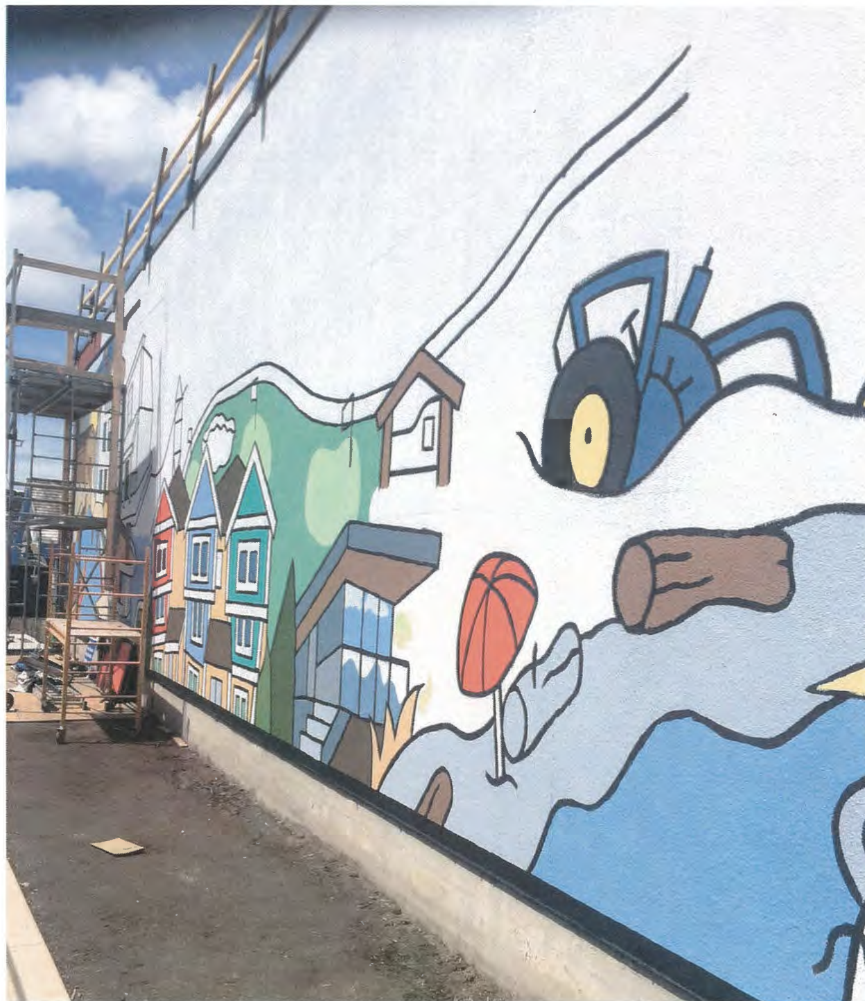
Mural being installed on Telus Building on 48 Avenue
