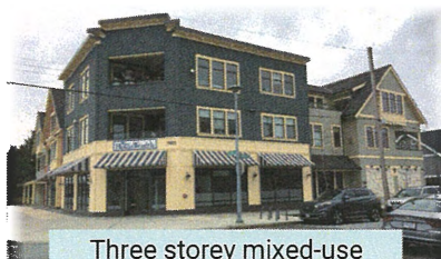
Three storey mixed-use building in Surrey
