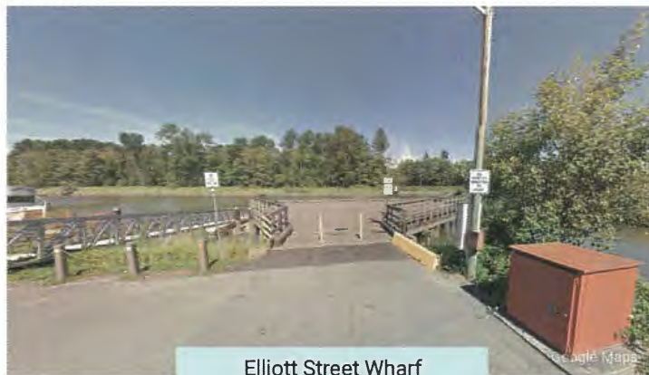
Elliott Street Wharf 5000 Chisholm Street
