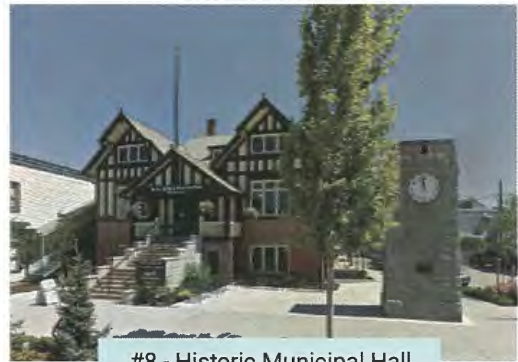
#8 - Historic Municipal Hall
