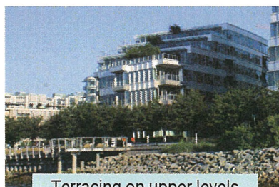
Terracing on upper levels of taller buildings
