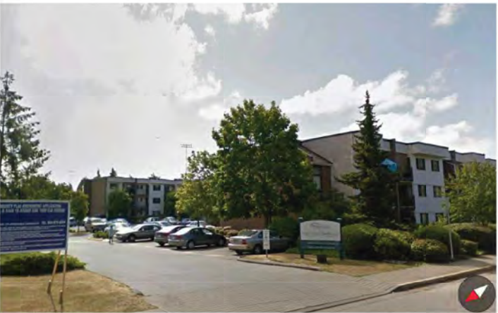
S2. EXISTING RESIDENTIAL RENTAL BLDG ON SITE, TO BE DEMOLISHED
