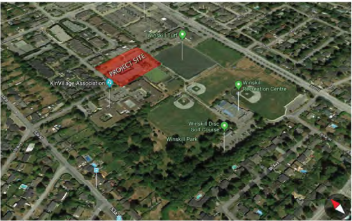
A1. SOUTH-WEST AERIAL VIEW
