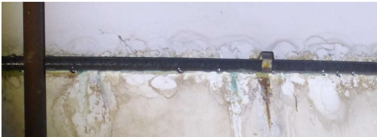
Condensation of water line in the mechanical room
