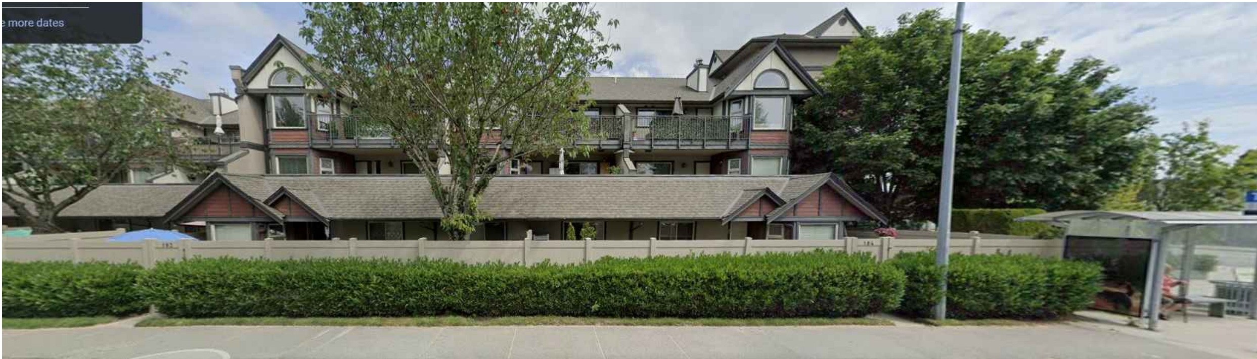
M) VIEW FROM LADNER TRUNK RD. (LOOKING NORTH)
