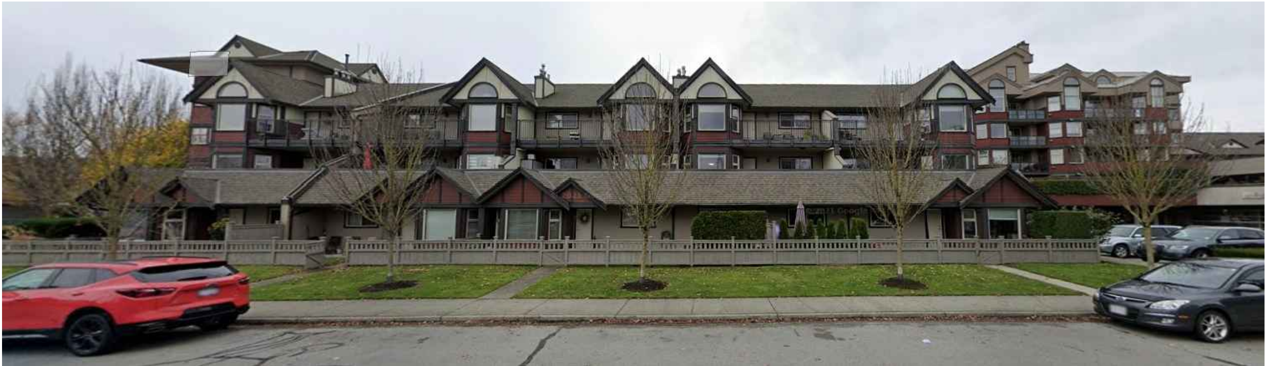
K) VIEW FROM 53 STREET (LOOKING WEST)
