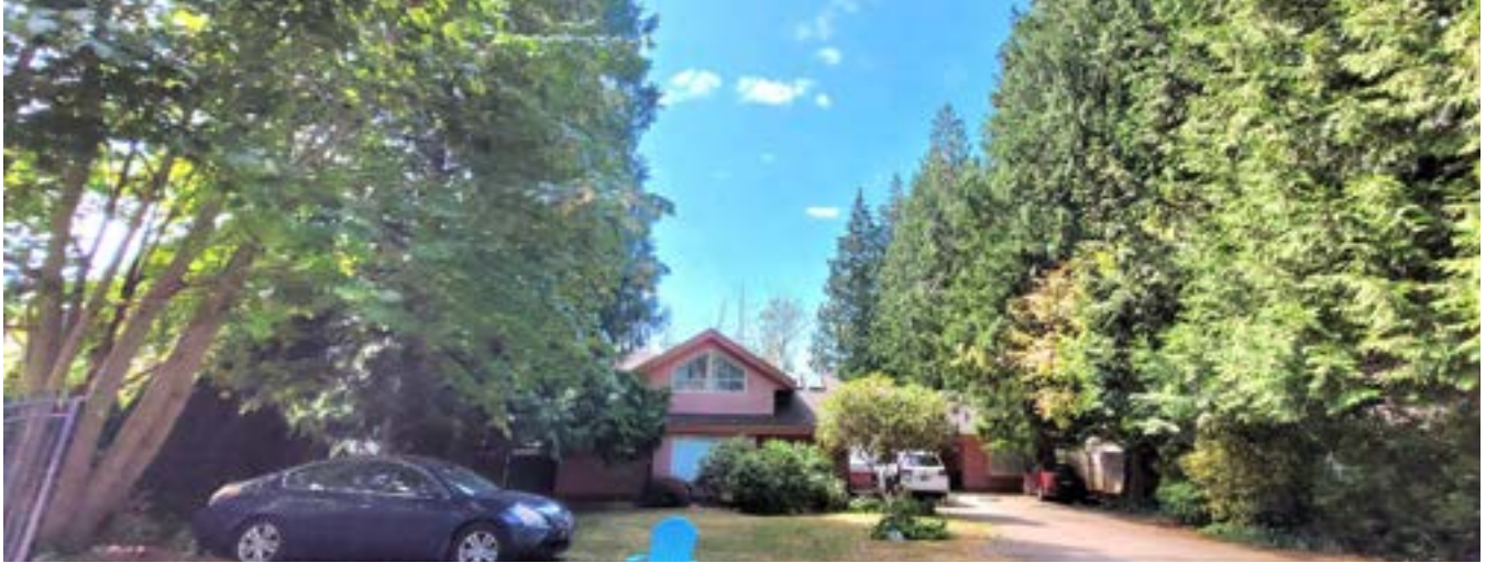
Photo 19 - Facing towards the southern section of the property and looking at the existing building
