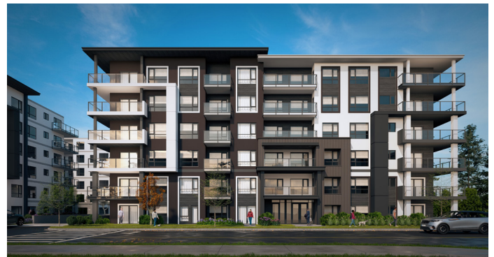
View from 90 Avenue, Lot 1 Facing South
