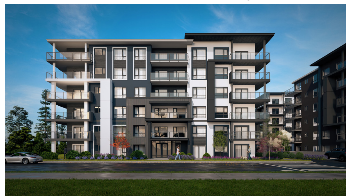
View from 90 Avenue, Lot 2 Facing South
