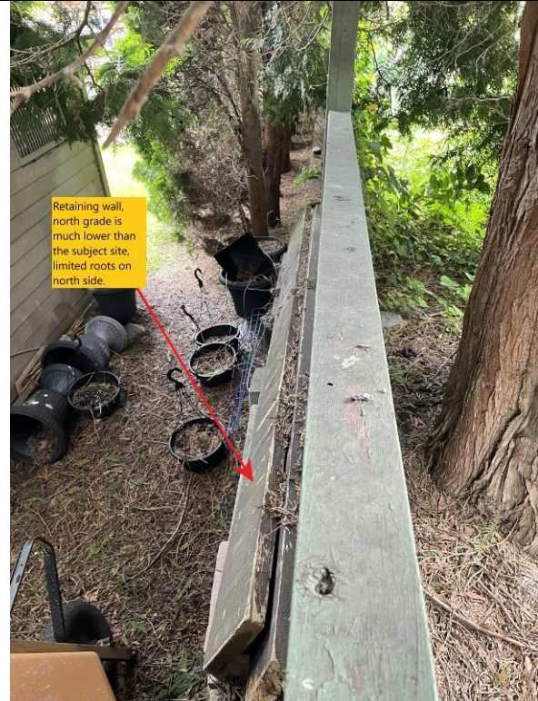
Photo 31: Retaining wall on north side of trunk, limited roots on neighbour's property.
