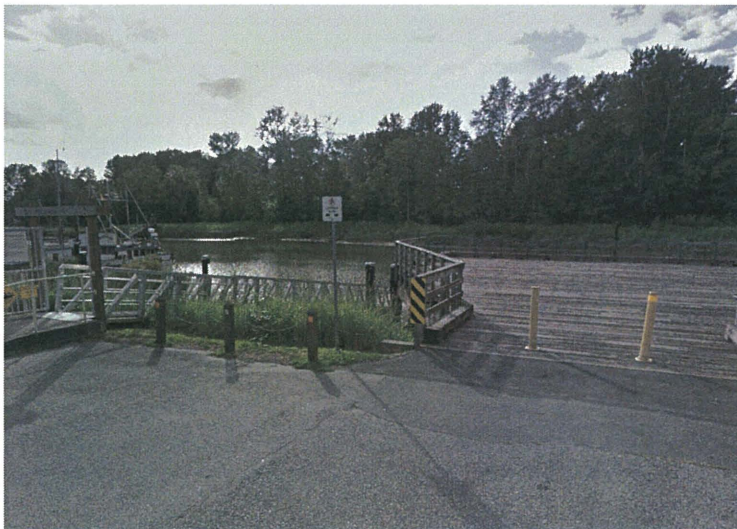
Elliott Street Wharf
