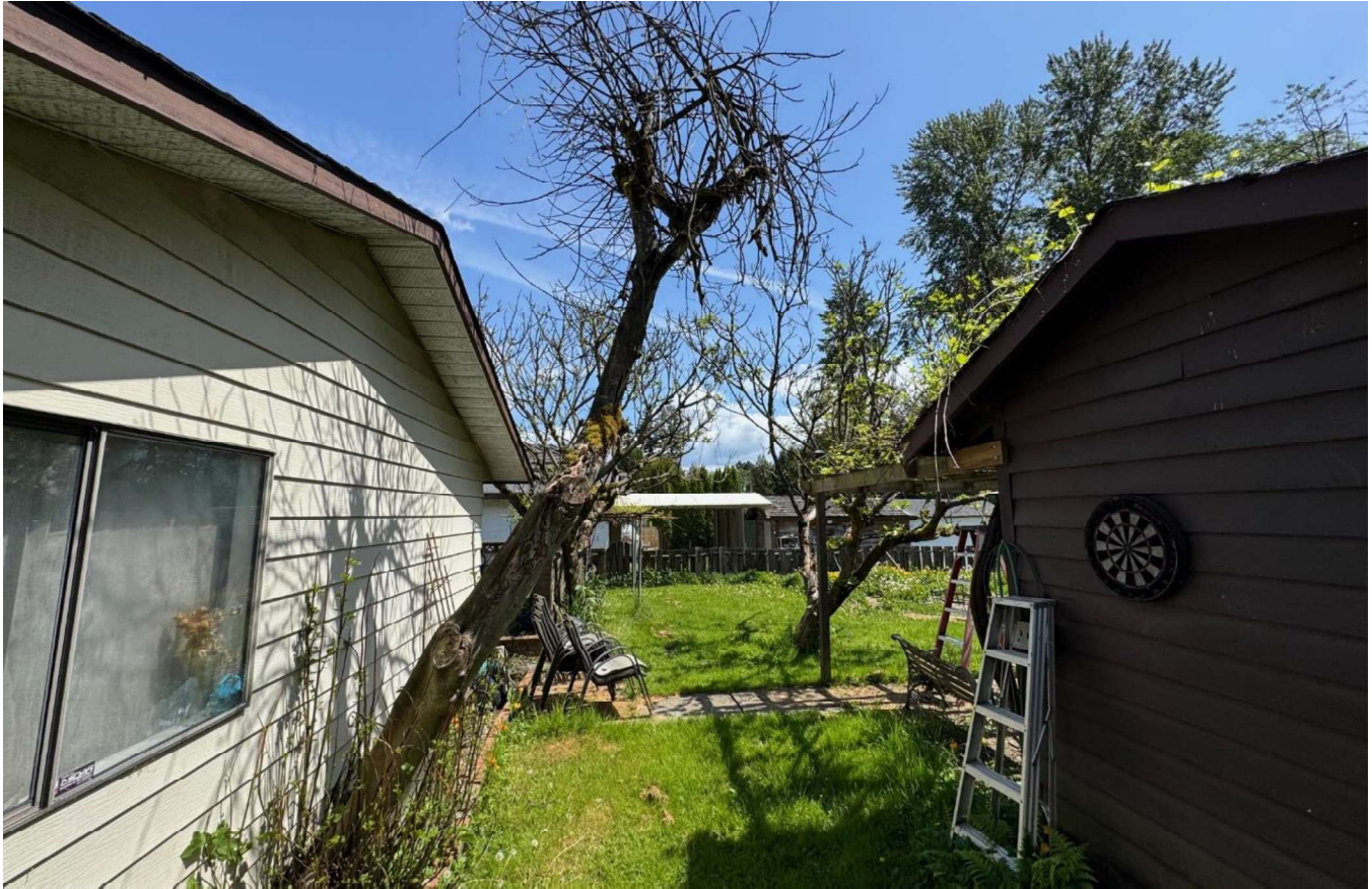
Photo 5 - Facing towards on-site trees #83, #84, and #85
