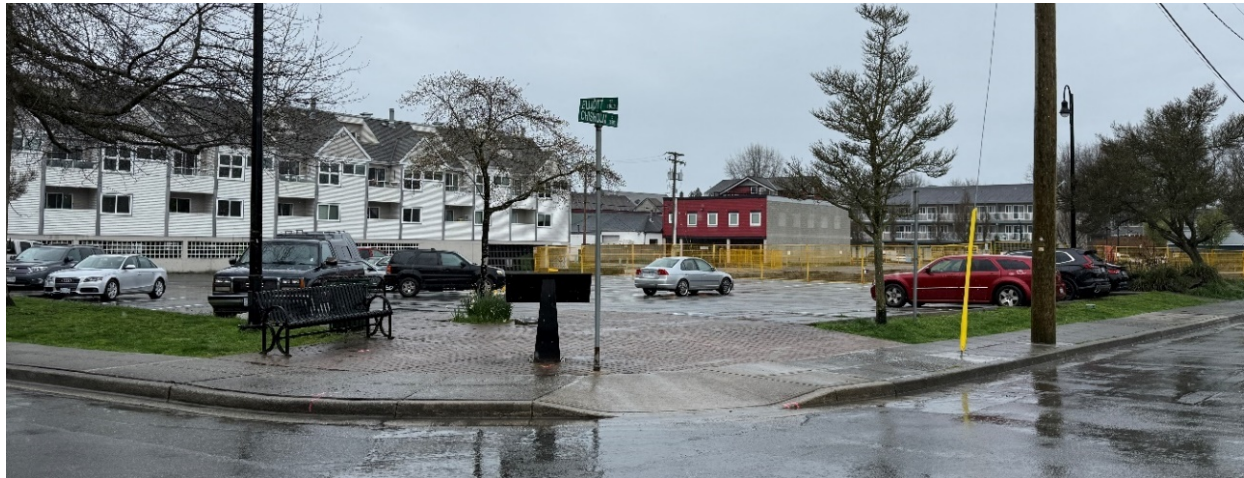
Figure 2 - Existing Conditions with Demolition in Progress
