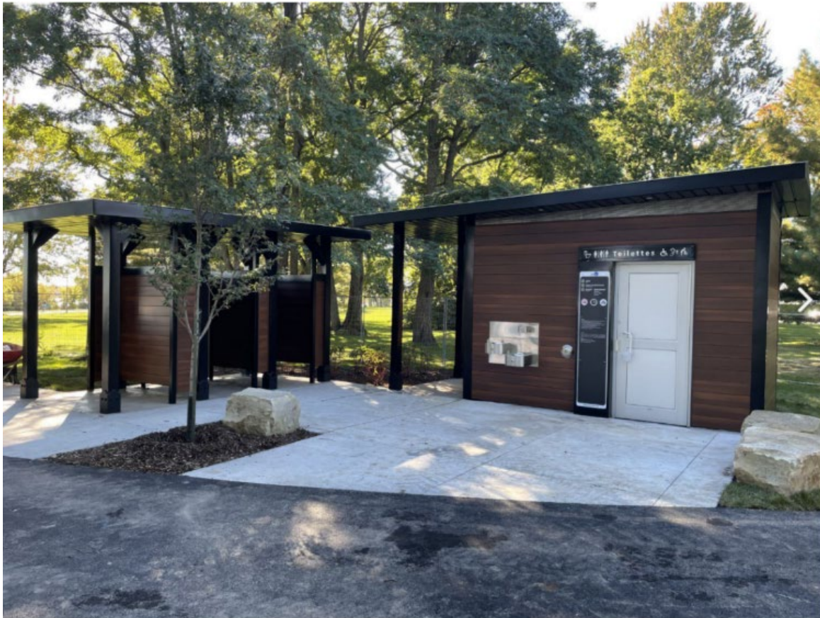
Figure 24 - Self-Cleaning Washrooms and Change Stalls - Park des Rapides, Montreal
