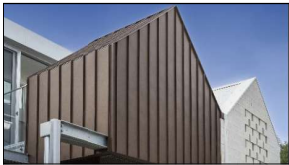
4. Standing Seam metal cladding Color to Match: Unicote Dusty coal
