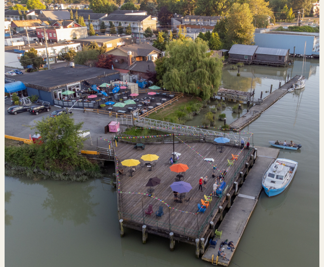
Ladner Village's Elliott Street Wharf
