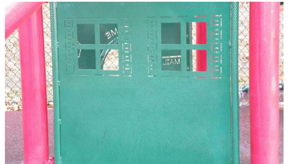
Steel Window Panel
